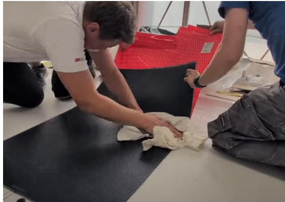
Fig. 19 - Pressing down the panel with a cloth
