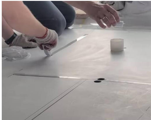
Fig. 16 - Primer applied on smooth surface
