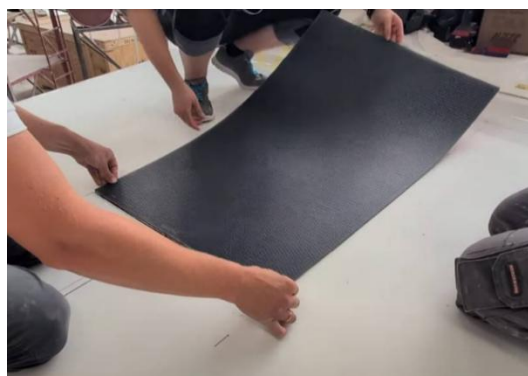
Fig. 17 - Placing panel in the desired location
